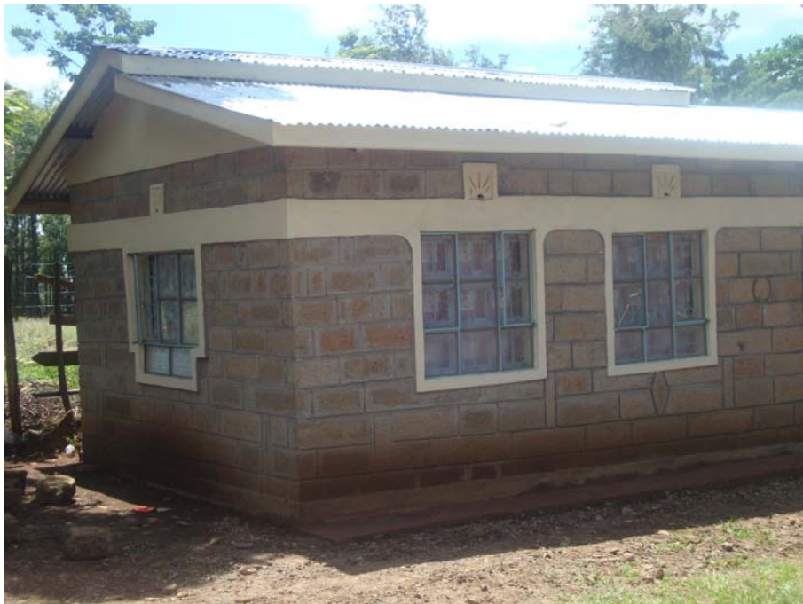
JKMC Office and Hall
